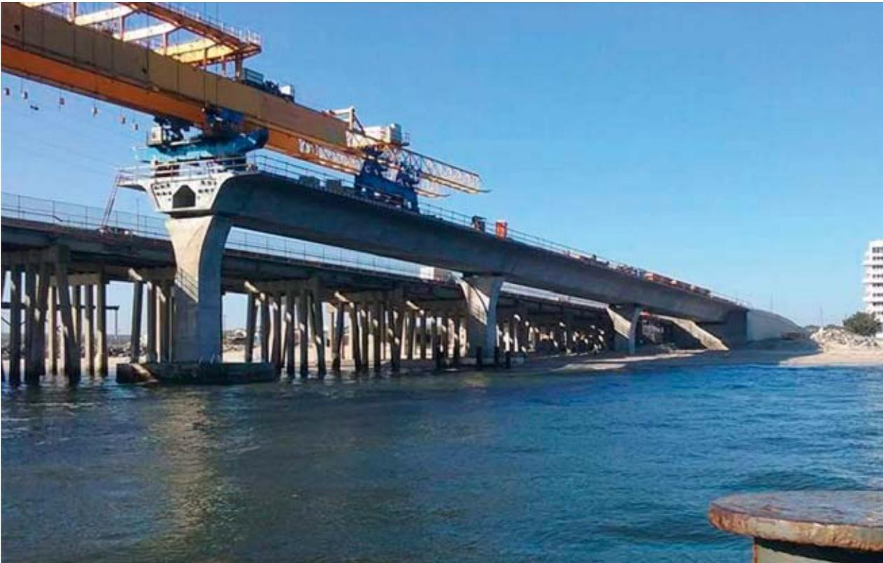
Corrosion had made replacement of the Lesner Bridge a necessity and the twin segmental structures of the new crossing now span Chesapeake Bay in the City of Virginia Beach, Virginia.
