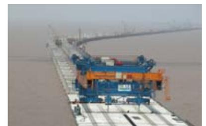
A state-of-the-art launching girder nicknamed Dennis has been developed by Deal to meet the demanding equipment requirements of a motorway scheme in Auckland
