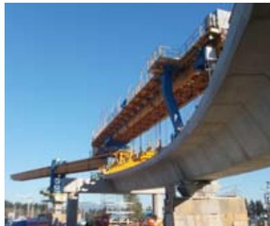
The 'hinged' feature of the equipment enabled a single launching truss to be used for the entire section of elevated line, with little disruption to the local traffic and neighbourhoods.
