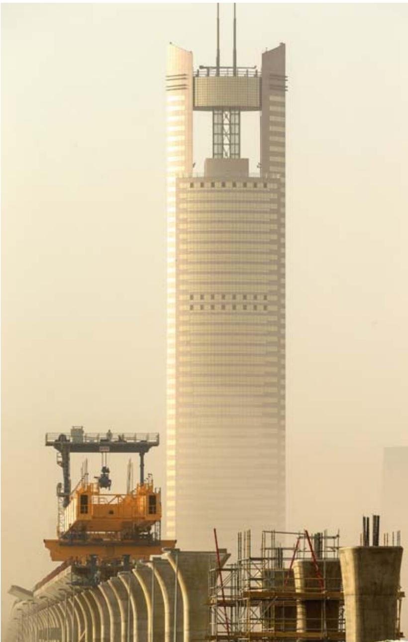
**The span-by-span method is being used to achieve high erection rates in the construction of the elevated sections of two metro lines**
