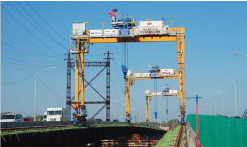
A special gantry crane, given the code name 'G19', has been designed by Deal for the reconstruction of the Moses Wheeler Bridge linking Stratford and Milford in Connecticut, USA.
