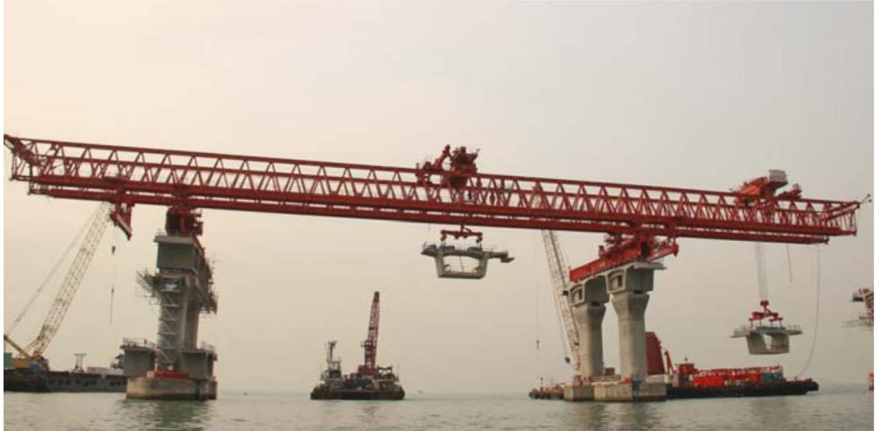
**The 'Red Dragon' has returned to bridge-building after a few years of inactivity. The distinctive launching girder is being used to construct prefabricated viaducts as part of a major bridge and tunnel project that will connect the cities of Hong Kong, Zhuhai and Macao on the Pearl River Delta**
