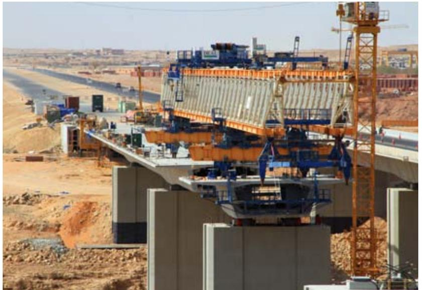
equipment that was already available and almost ready to use. Fabrication of the precast elements was able to start just four months after the award of the contract, thanks to the work done during the 're-engineering' stage to prepare and ship to site all of the specially modified prefabrication equipment.
