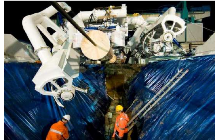
Trenching machine, Caspian Sea, Kazakhstan
