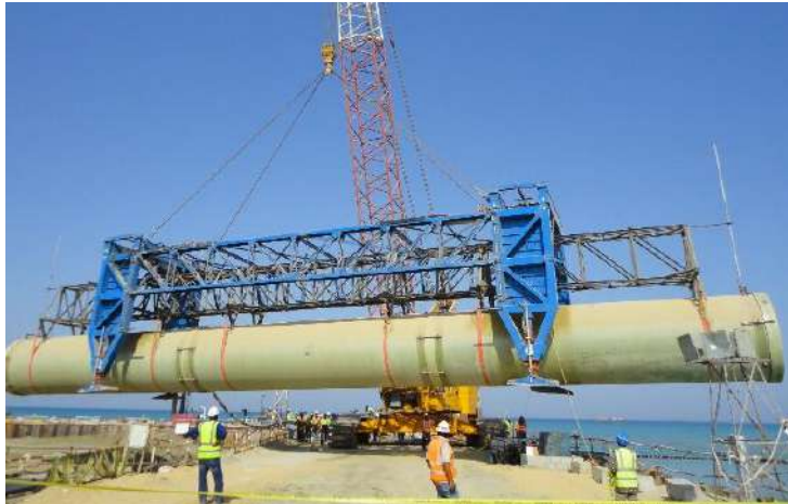
Underwater spreader beam, El Ain Sokhna, Egypt
