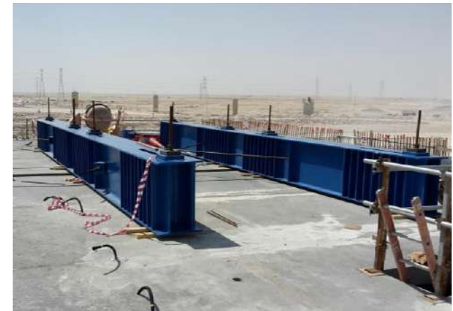
Alignment beams for Orbital Road, Doha, Qatar
