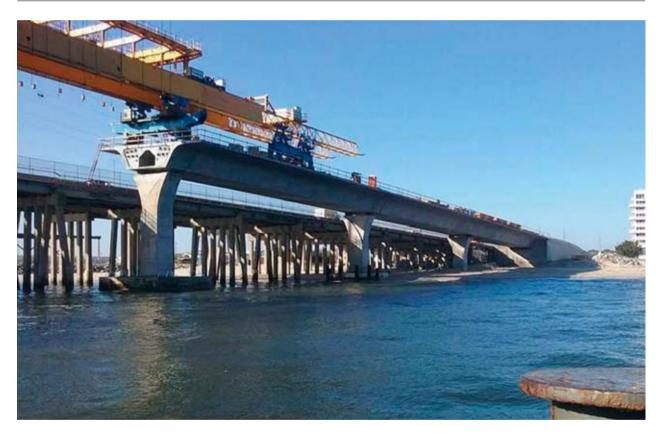
orrosion had made replacement of the Lesner Bridge a necessity and the twin segmental structures of the new crossing now span Chesapeake Bay in the City of Virginia Beach, Virginia.
