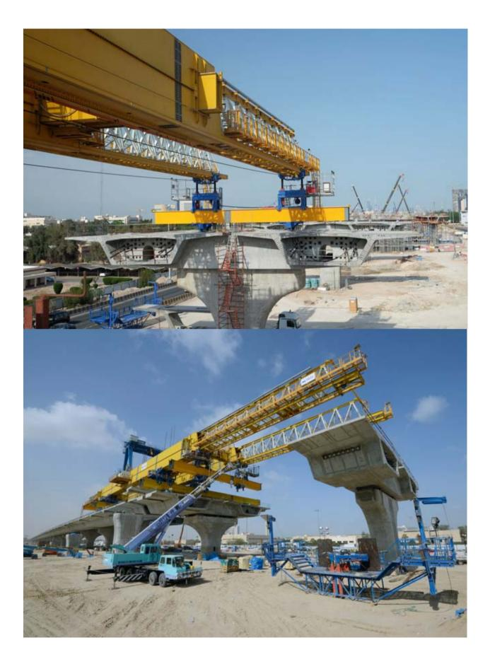
One of Kuwait's key infrastructure and road development projects - Use of precast segmental erection methods to construct 395,000sqm of viaducts - Design life of 100 years In order to increase the production rate and to optimise the quantities of materials (rebar and tendons), Deal proposed an alternative construction method for part of the project
