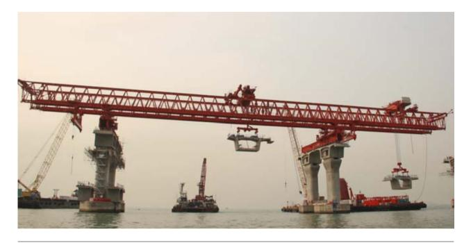
The 'Red Dragon' has returned to bridge-building after a few years of inactivity. The distinctive launching girder is being used to construct prefabricated viaducts as part of a major bridge and tunnel project that will connect the cities of Hong Kong, Zhuhai and Macao on the Pearl River Delta
