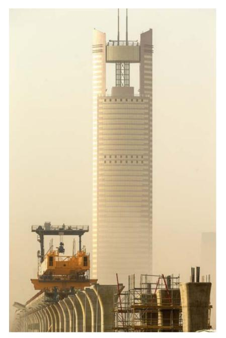
The span-by-span method is being used to achieve high erection rates in the construction of the elevated sections of two metro lines
