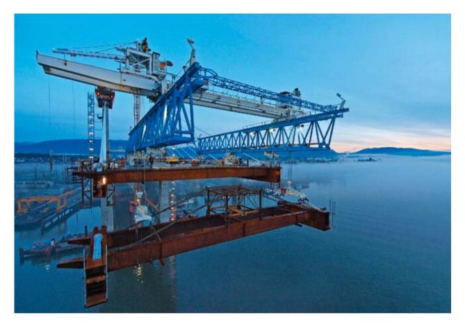
Bridge. The through-arch bridge in Long Beach, California, was built in 1968 across Cerritos Channel to provide a link to Terminal Island. The old bridge has recently been encountering structural and maintenance problems, so the Port Authority decided to replace it with a new cable-stayed bridge with 61m of vertical clearance. The new bridge will allow access into the port for the tallest container ships and will be the first long-span cable-stayed bridge in California.
