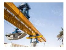
on a production cycle that starts in the precast yard, where the segments are manufactured, and ends with the erection equipment that physically builds the bridge. All the items of equipment required for the entire process - 29 precasting moulds, four gantry cranes, five launching girders and four lifting frames – have been provided by Deal. Deal has to design, manufacture and deliver all of the equipment in accordance with a strict schedule - a huge
