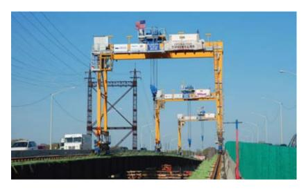
A special gantry crane, given the code name 'G19', has been designed by Deal for the reconstruction of the Moses Wheeler Bridge linking Stratford and Milford in Connecticut, USA.
