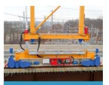
A special gantry crane moving along a curved alignment
